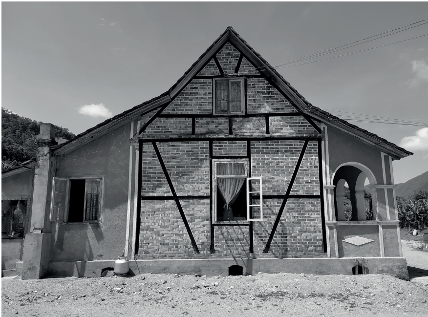
Figure 9. A house in the Hungarian Cultural Route. Source: by the author (2022)
